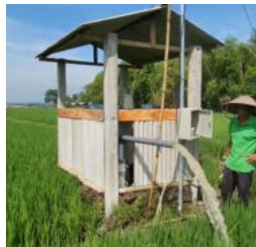
The completed shelter
