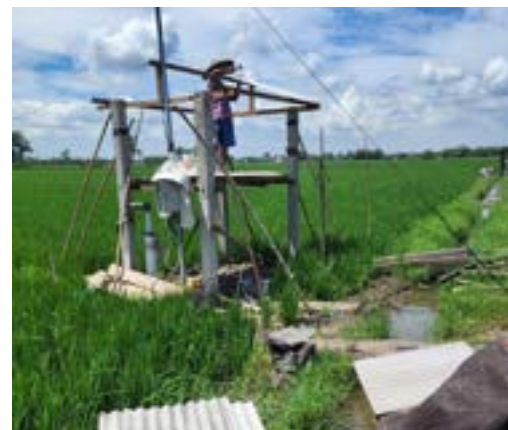
Building the shelter around the pump
