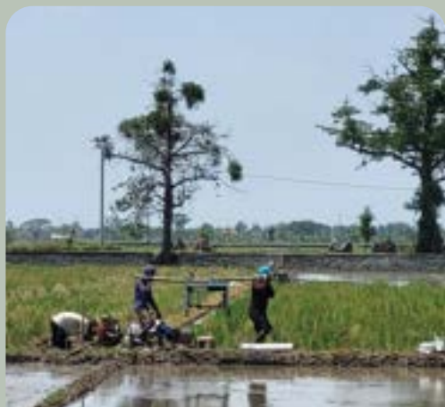
Excavating for the submersible water pump
